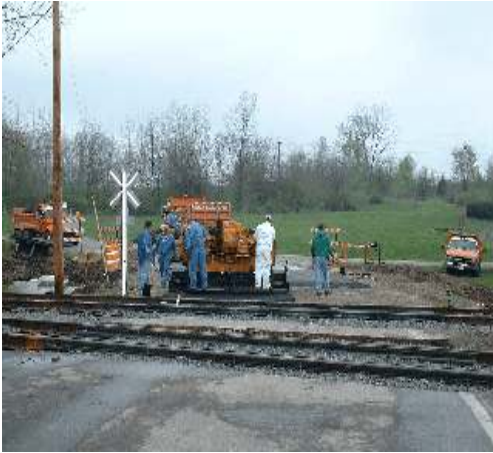
Paving at Culvert installation on Muzzy
