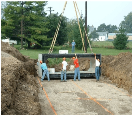
Installing Box culvert on Mutual Union Road.
