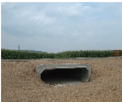
Culvert installation on East Kingscreek Road
