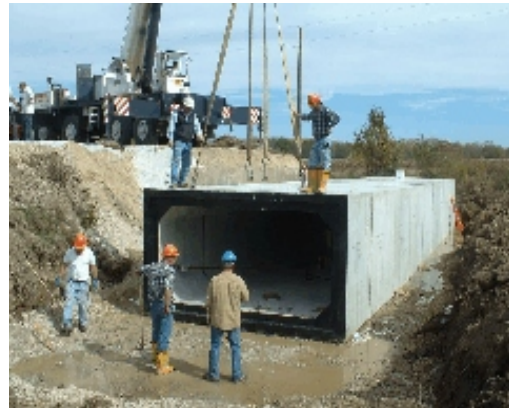
Installing box culvert on Elm Tree Road.
