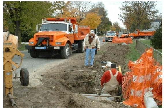
Storm sewer installation in Millerstown
