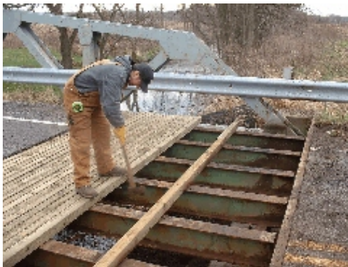
Deck Repair on Kennard-Kingscreek Road
